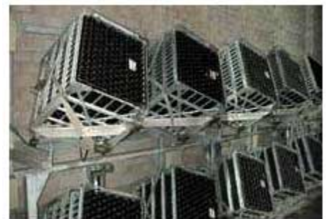
Mounting the gyropalettes on the wall in banks provides riddling consistency in a synchronous operation, accompanied by flashing lights and sirens to warn workers out of harm's way.
